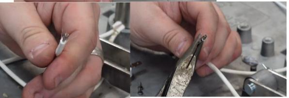
Strip and crimp the new connector for each wire.
